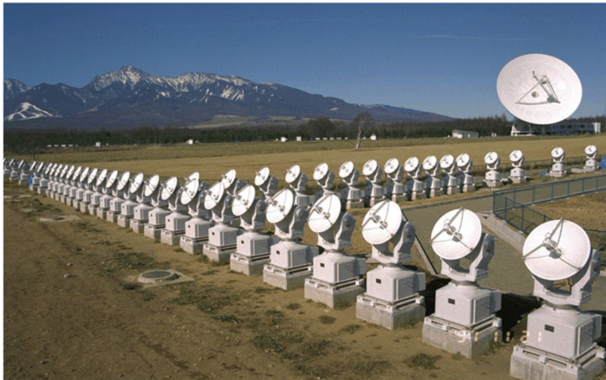
Fig. 1.10 The Nobeyama Radioheliograph (NoRH) in Japan, consisting of 84 parabolic antennas with 80 cm diameter, arranged in two arms, one with a length of 490 m in east/west direction, the other with a length of 220 m in north-south direction. First observations were made in April 1992, and are continued already over 25 years (Credit: NRO/NAO, Japan)
